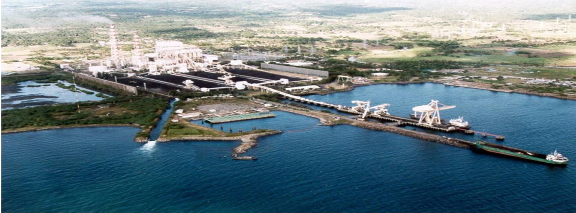
Figure 3: Aerial view of the Power Plant
